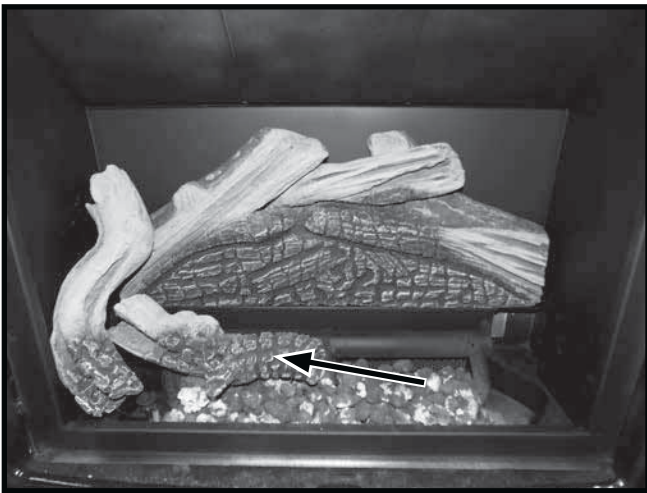
Figure 49: 3rd log placement.
