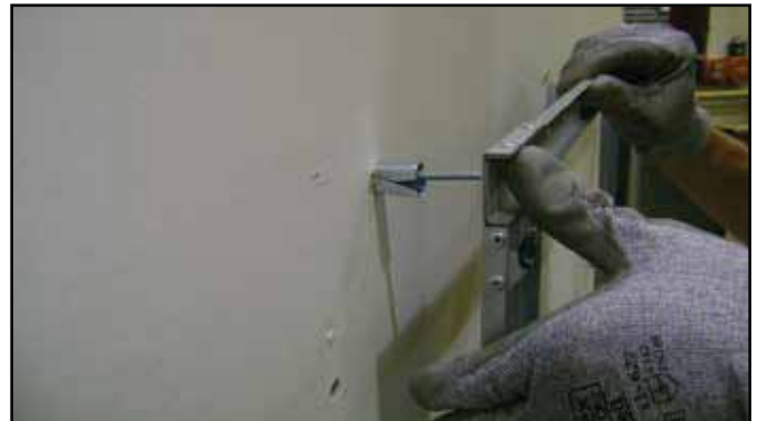
Figure 5 Installing Anchors in Hollow Wall
