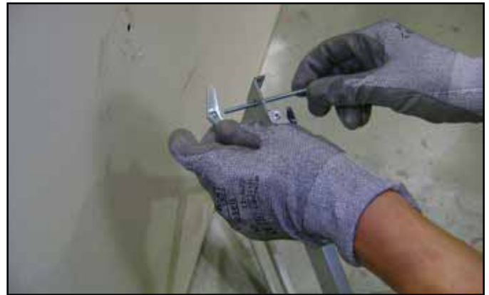
Figure 4 Toggle Bolt Installation through Mounting Bracket
