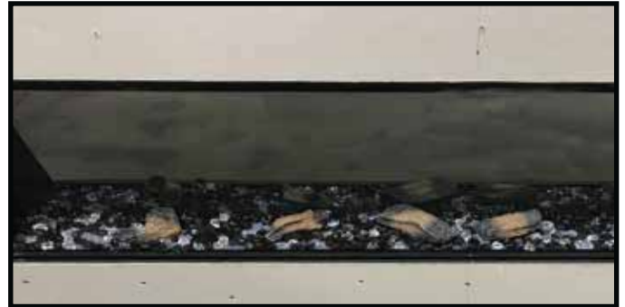
Figure 4.10 Media and Small Logs Installation
