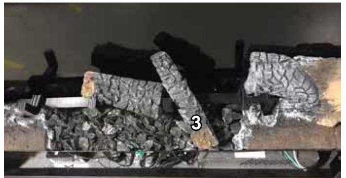
Figure 4.24 Install Log #3
