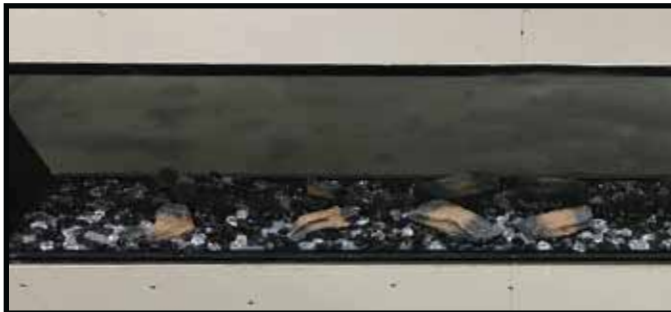
Figure 4.12 Media and Small Logs Installation
