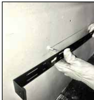
Figure 4.5 Installing Anchors in Hollow Wall
