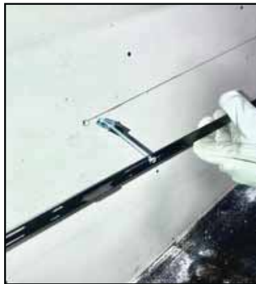
Figure 4.4 Toggle Bolt Installation through Mounting Bracket
