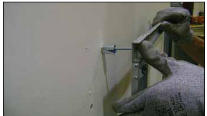
Figure 4.11 Installing Anchors in Hollow Wall
