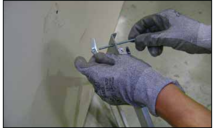
Figure 4.10 Toggle Bolt Installation through Mounting Bracket
