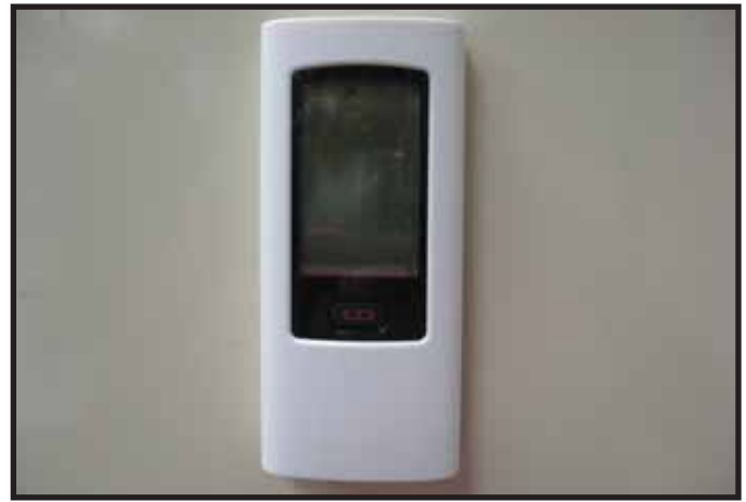
Figure 4.4. Mounting Remote Control Housing
