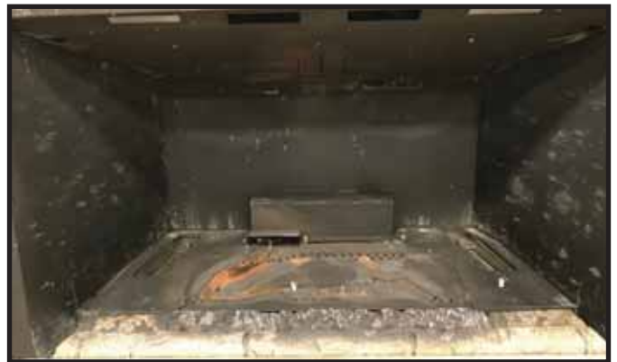
Figure 3 Base Refractory Installed
