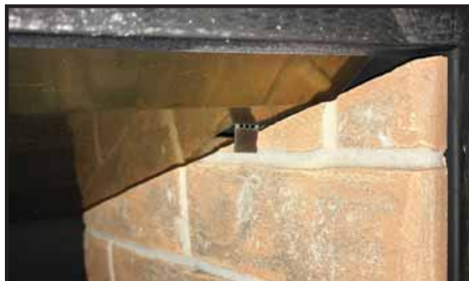
Figure 7 Right Refractory Handbend Tab
