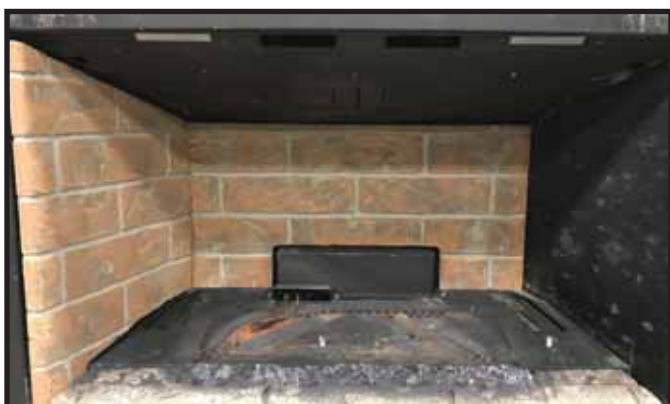
Figure 5 Left Refractory Installed
