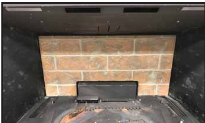
Figure 4 Back Refractory Installed
