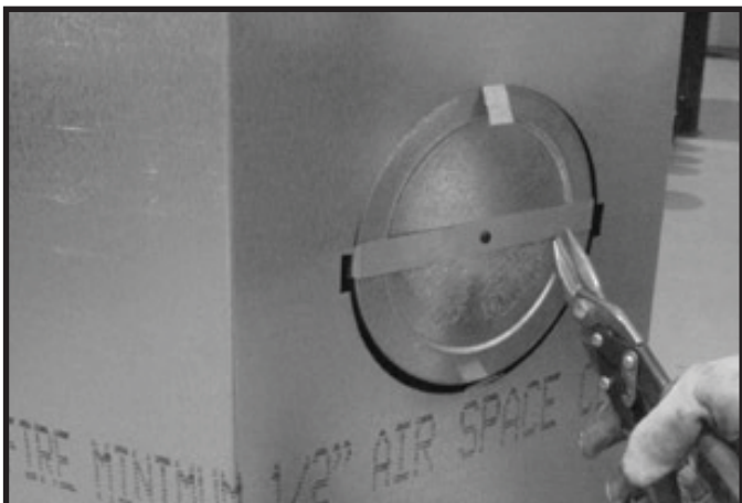
Figure 6.13 (Generic Fireplace Shown) Cut the metal retaining band and fold the sides out.
