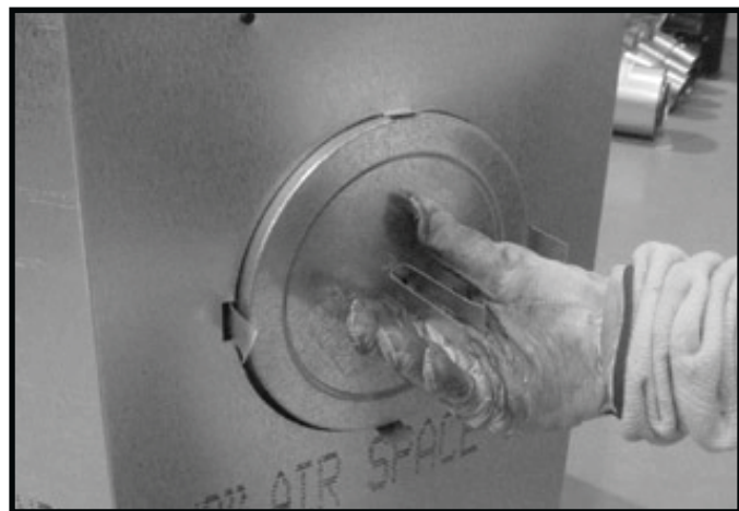
Figure 6.10 (Generic Fireplace Shown) Fold the center parts of the retaining band out and use to remove the seal cap.
