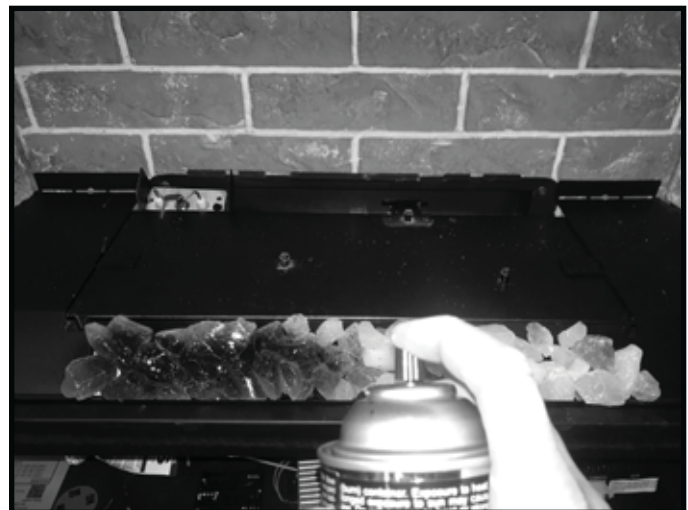
Figure 11.2 Paint Teco-Sil
