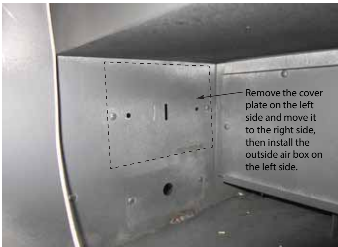
Figure 3.14 Remove Cover Plate (Left Side)
