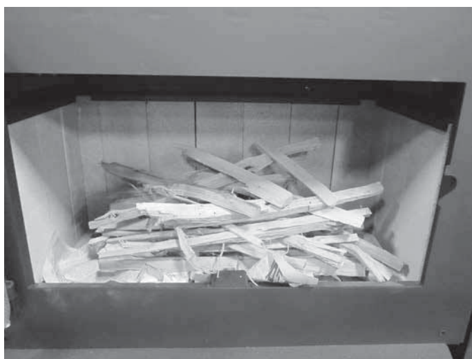
Figure 3.21 Placing Kindling
