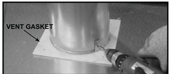
**Figure 6.11 (Generic Fireplace Shown)** To attach the first section of vent pipe, make sure to use the vent gasket in the manual bag to seal between the first vent component and the outer fireplace wrap. Seal with four screws or caulk with a minimum of 300 °F continuous exposure rating may be used to hold the part in place.
