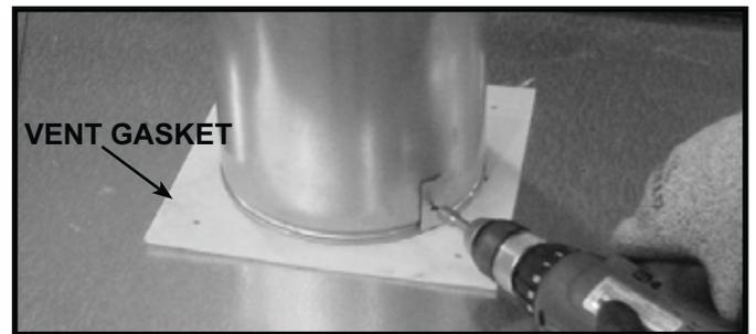
**Figure 6.6 (Generic Fireplace Shown)** To attach the first section of vent pipe, make sure to use the vent gasket in the manual bag to seal between the first vent component and the outer fireplace wrap. Seal with four screws or caulk with a minimum of 300 °F continuous exposure rating may be used to hold the part in place.
