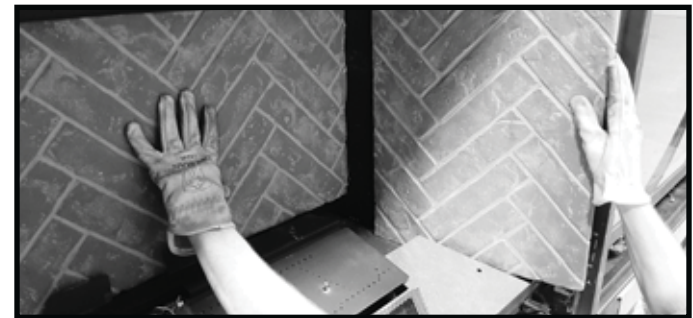
Figure 11.3 Install Side Refractory Panel (Right Side Shown)
