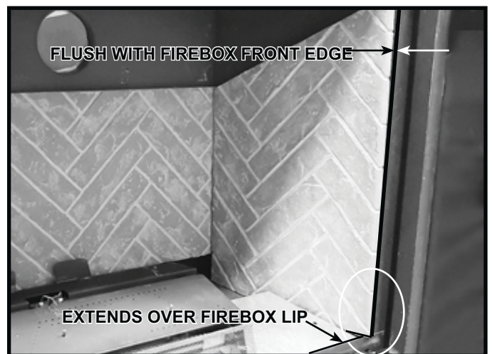
Figure 11.4 Side Refractory Panel Installed (Right Side Shown)
