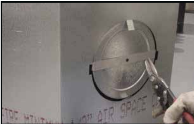
Figure 6.13 (Generic Fireplace Shown) Cut the metal retaining band and fold the sides out.
