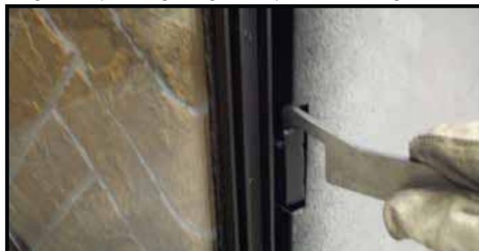
Figure 11.7. Securing Side Glass Clips
