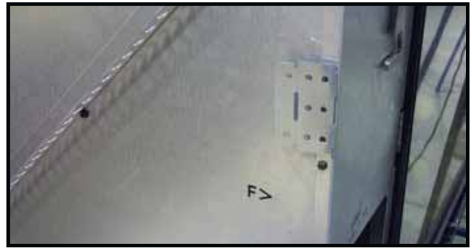
Figure 6.3 Side Nailing Tab in Shipping Position
