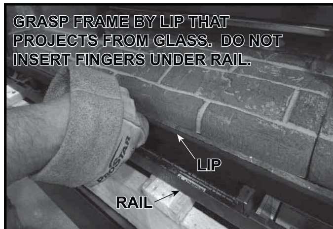
Figure 11.6. Installing Glass
