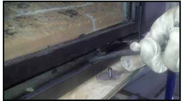
Figure 11.2. Glass Clip Tool Location
