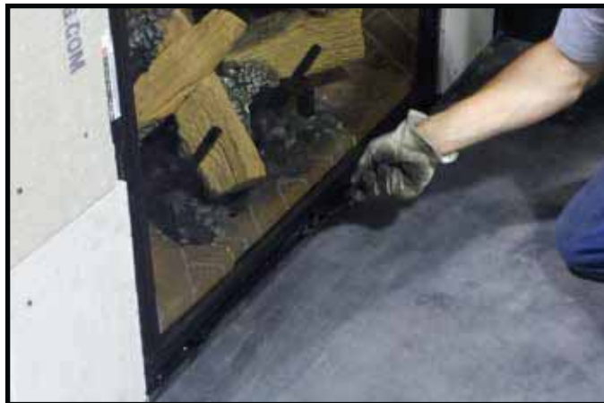
Figure 11.8. Securing Bottom Glass Clips
