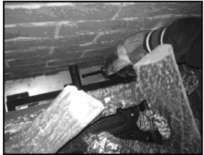
Figure 9.1. Air Shutter Location
