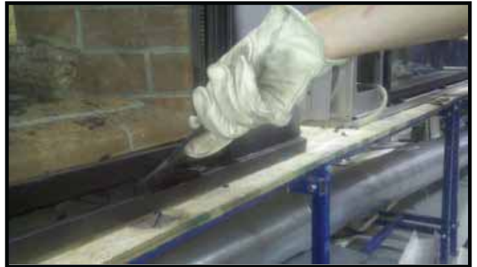
Figure 11.3. Inserting Glass Clip Tool
