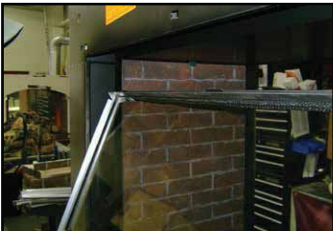
Figure 11.2 Initial Positioning of Frame into Opening.
