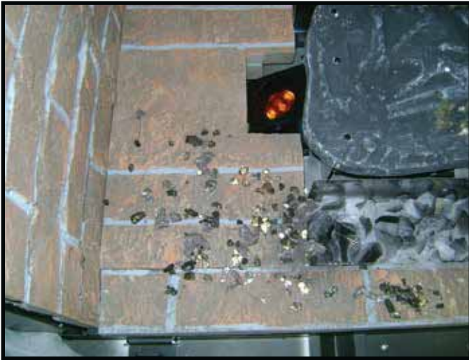
Figure 11.17 Ember Placement on Base Refractory
