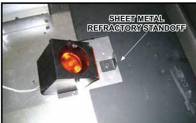
Figure 11.13 Accent Light Bulb Installation Completed
