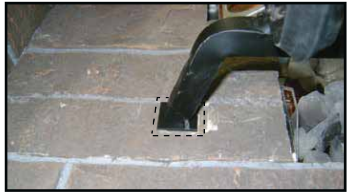
Figure 3. Grate leg placement.
