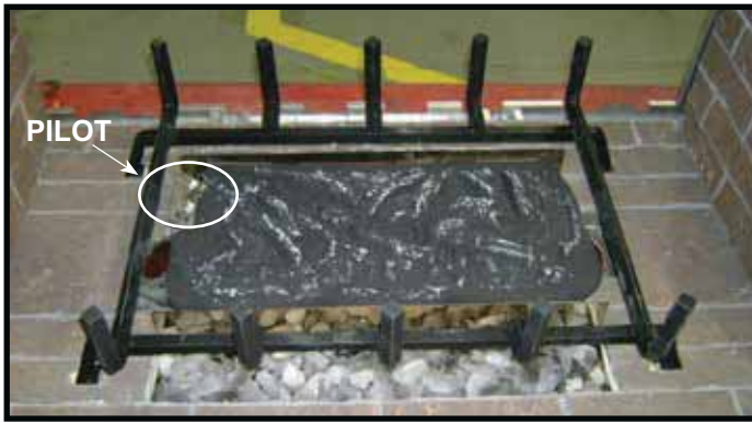
Figure 2. Burner and grate from front.
