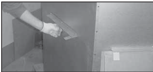
Figure 3.7 Bending Refractory Shipping Tabs Back Down
