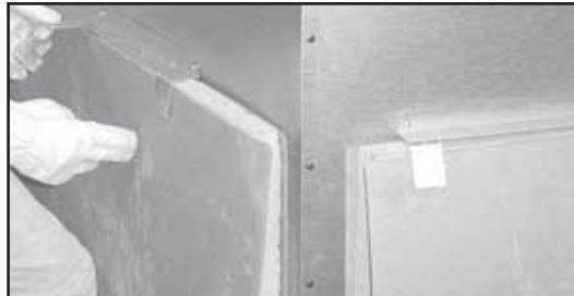
Figure 3.6 Unpacking Back Refractory
