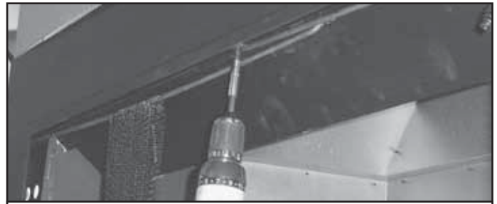
Figure 3.9 Removing the Screen Rods
