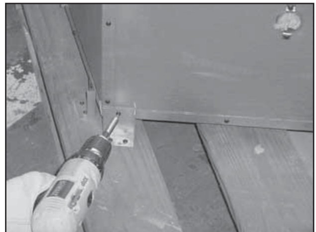
Figure 3.12 Removing Shipping Brackets
