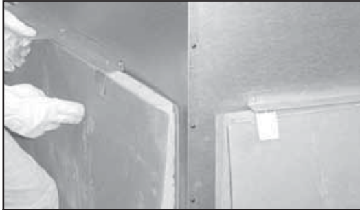
Figure 3.6 Unpack Back Refractory
