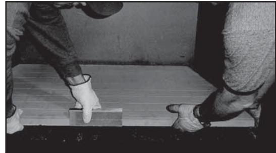
Figure 3.10 Lifting Out Hearth Stone
