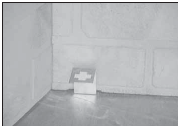
Figure 8.8 Grate Retaining Bracket in Place
