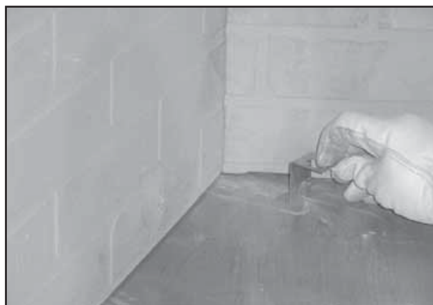
Figure 8.7 Slide Grate Retaining Bracket into Notch
