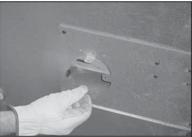
Figure 3.19 Bending Tabs on Outside Air Kit Collar
