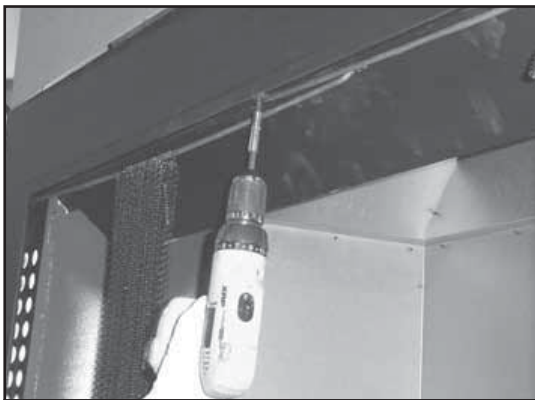
Figure 3.8 Remove Screen Rods
