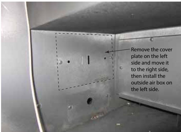
Figure 3.14 Remove Cover Plate (Left Side)
