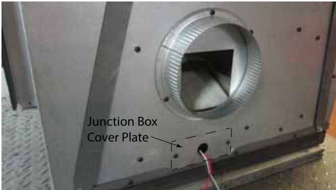
Figure 4.1 Junction Box Cover Plate
