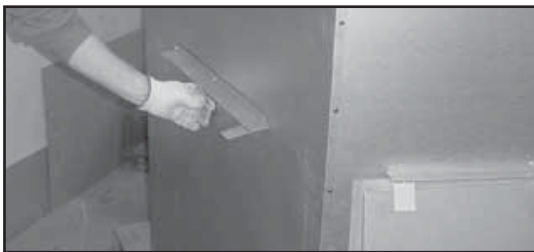
Figure 3.7 Bending Refractory Shipping Tabs Back Down
