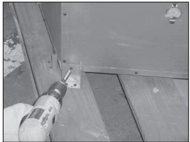
Figure 3.12 Removing Shipping Brackets
