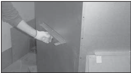
Figure 3.7 Bend Refractory Brackets Back Down
