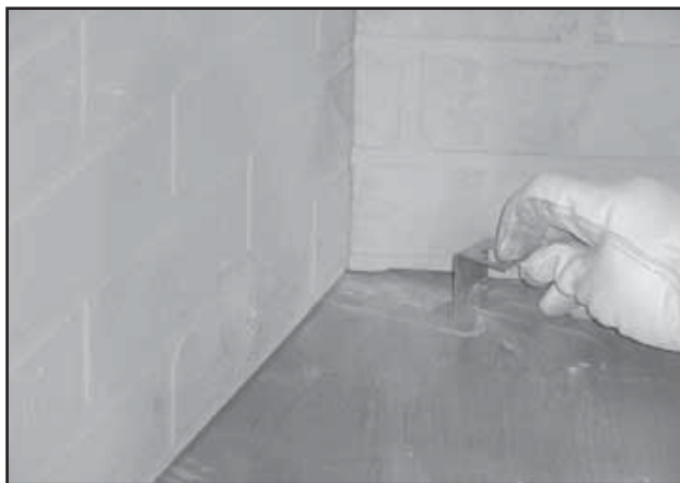
Figure 8.7 Slide Grate Retaining Bracket into Notch
