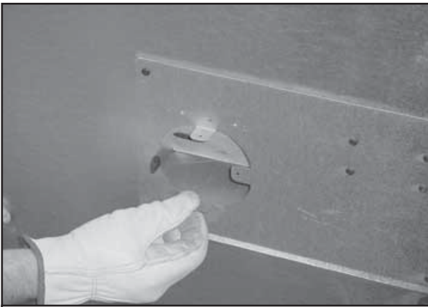
Figure 3.18 Bending Tabs on Outside Air Kit Collar
