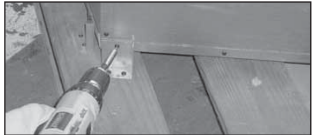
Figure 3.11 Removing Shipping Brackets
