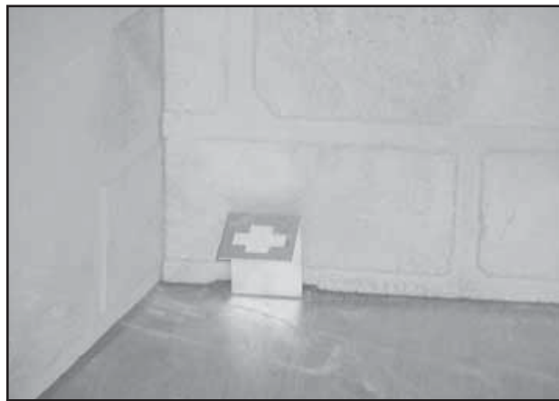
Figure 8.8 Grate Retaining Bracket in Place
