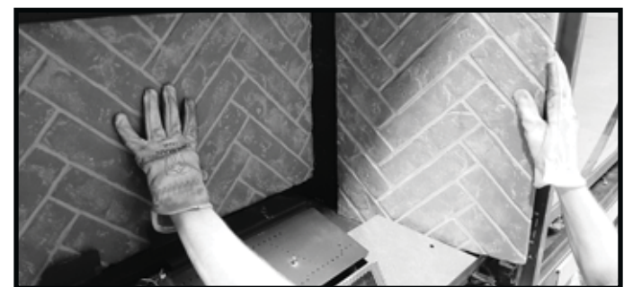
Figure 11.3 Install Side Refractory Panel (Right Side Shown)
