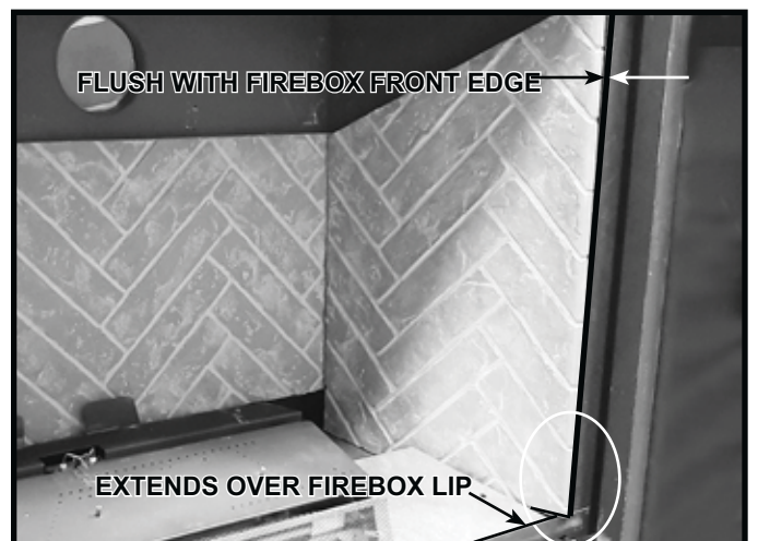
Figure 11.4 Side Refractory Panel Installed (Right Side Shown)
