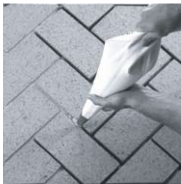
Figure 25 - Grouting Brick
