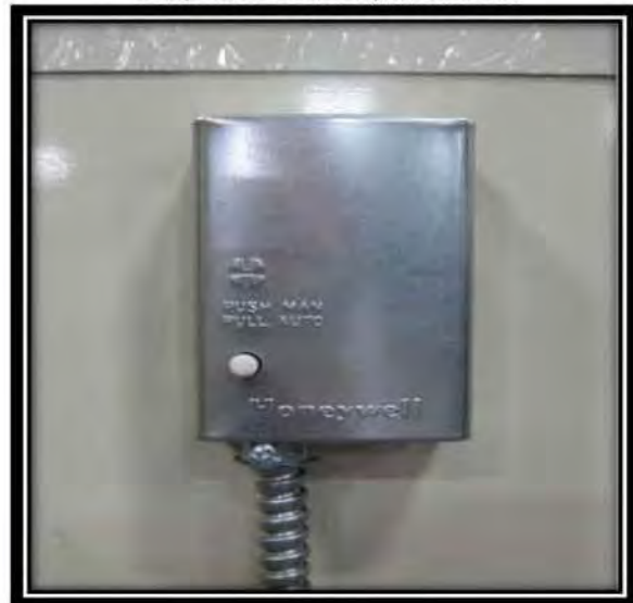
Fan/Limit Control, Mounted
