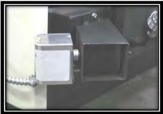
Automatic Draft Tube with Damper Control Motor
