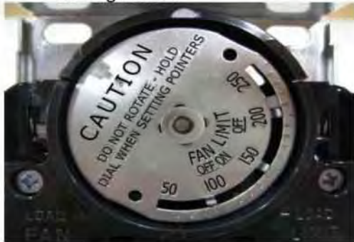
Fan/Limit Control Settings
