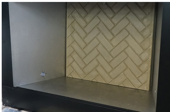
Install Back Refractory Figure 48
