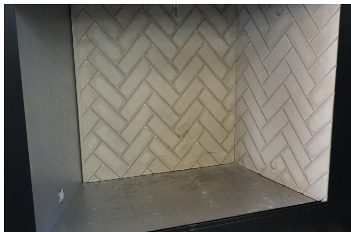
Install Right Side Refractory Brick Liner Figure 50
