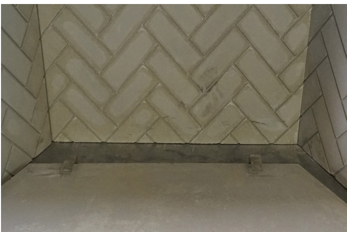
Install Hearth Refractory With Grate Retainers Figure 52
