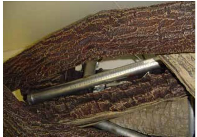
**Figure 25A - Installing Back Top Log, Top View**
