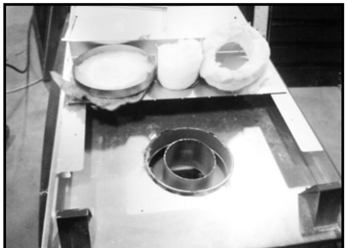
Figure 6.5 Remove and discard the seal cap, insulation donut, insulation plug, and the insulation basket. Attach the first vent section (it will snap into place). Slide the vent gasket onto the vent section and then, up against the appliance. Secure the vent gasket to the appliance with two self-tapping screws found in the manual bag. Note: The vent gasket can found in the manual bag.
