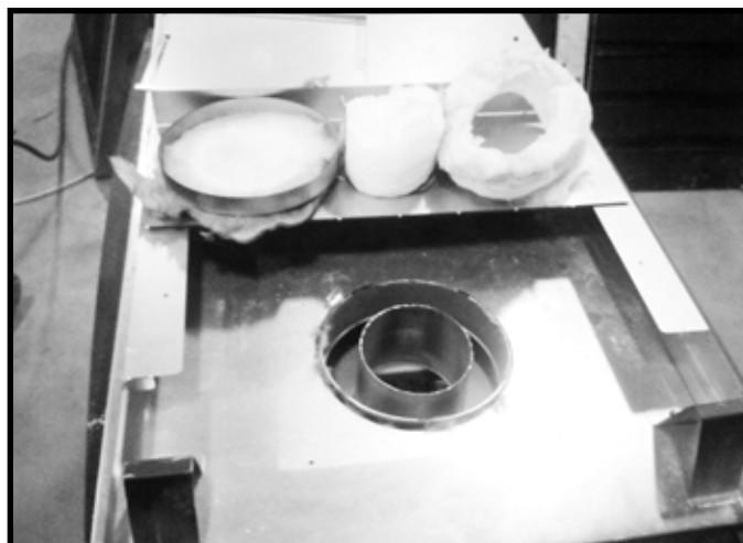
Figure 6.3 Remove and discard the seal cap, insulation donut, insulation plug, and the insulation basket. Attach the first vent section (it will snap into place). Slide the vent gasket onto the vent section and then, up against the appliance. Secure the vent gasket to the appliance with two self-tapping screws found in the manual bag. Note: The vent gasket can found in the manual bag.
