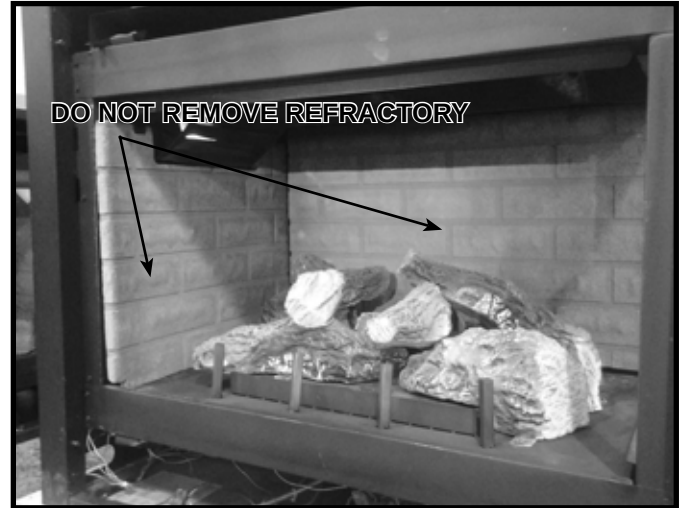
Figure 2.2 Do Not Remove Refractory
